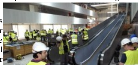
(Part of interior of new airport)
